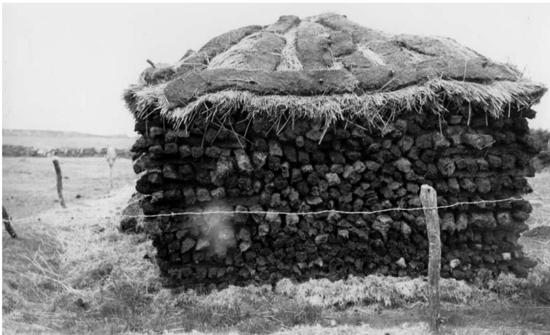
Fig 101 Rick built c 1940 on a turf stead at the cutting grounds, possibly Pridacoombe Downs, Altarnun (SX 164773). The stacked turves were cut with a turf iron and those holding down the rush thatch are skimmies (see also Fig 100). Note how the quoins are carefully bound in with overlapping turves and the rick's sides are sprung to protect it from the elements. The stead has been reused as the ditch has not been freshly cut. Grazing animals were kept at bay by the single strand barbed-wire fence. (From the archive of CK Croft Andrew, held at CCC HES)
