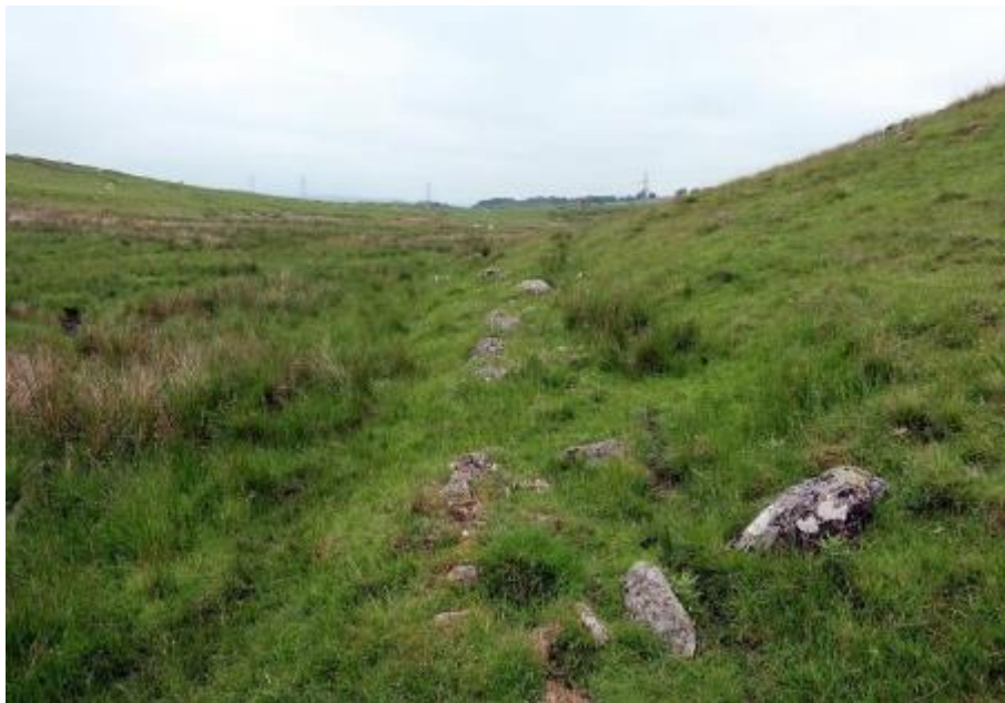
Covered aqueduct (P21, 2022 Report)
